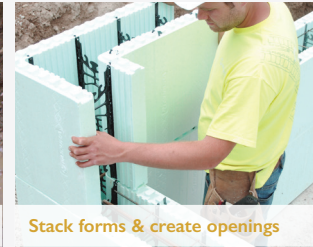
Place rebar in the walls
